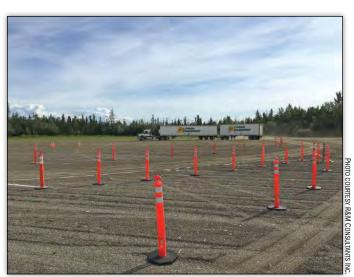
To assure the trucking industry that the roundabout could handle commercial vehicles of all sizes, R&M Consultants organized a truck trial and invited truckers to drive a full-sized mockup of the proposed design.
