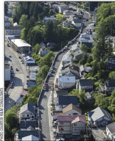
The finished Water Street Bridge project, seen from the air, includes new construction of a 1,000-foot-long hybrid concrete-steel trestle bridge system consisting of a 700-foot pile-supported concrete deck panels, 200-foot retaining wall on both sides with fill, and a 100-foot prestressed concrete deck bulb tee girder span.
