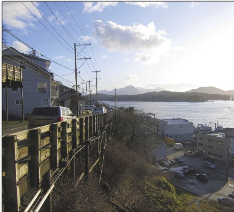
Utility lines that crisscrossed the road and were closely bundled along its length in this photo of the pre-demolition bridge. In order for construction work to proceed, an advanced utility relocation project rerouted transmission lines along alternate corridors. Utilities that remain were mostly relocated to below the bridge deck including the Ketchikan Public Utilities water, sewer, electrical power, TV and telephone.
