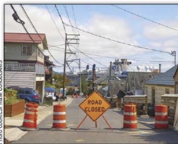
A section of the new bridge was closed in late June for the long-awaited ribbon-cutting and official opening. The photos show how tightly houses and utility lines are clustered along the road, which leads to the waterfront, where cruise ships are docked in the distance. Dawson Construction invented a piece of equipment, dubbed the panel launcher, that allowed placing 5-foot by 20-foot concrete panels into place in tight space.
